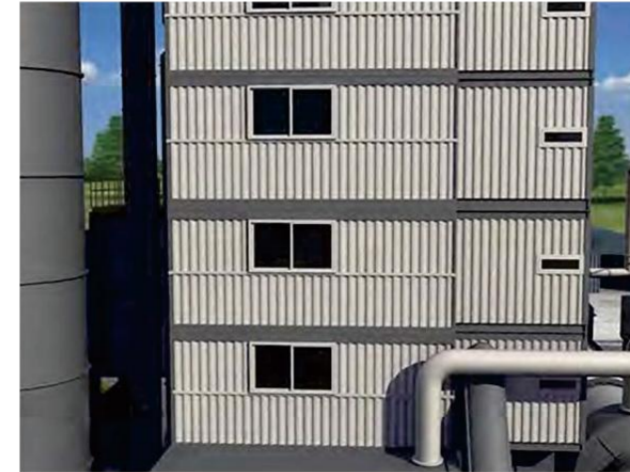
Enclosed mixing tower
